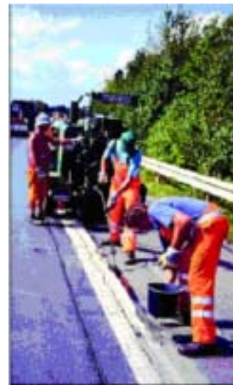
Risse in Asphalt füllen
