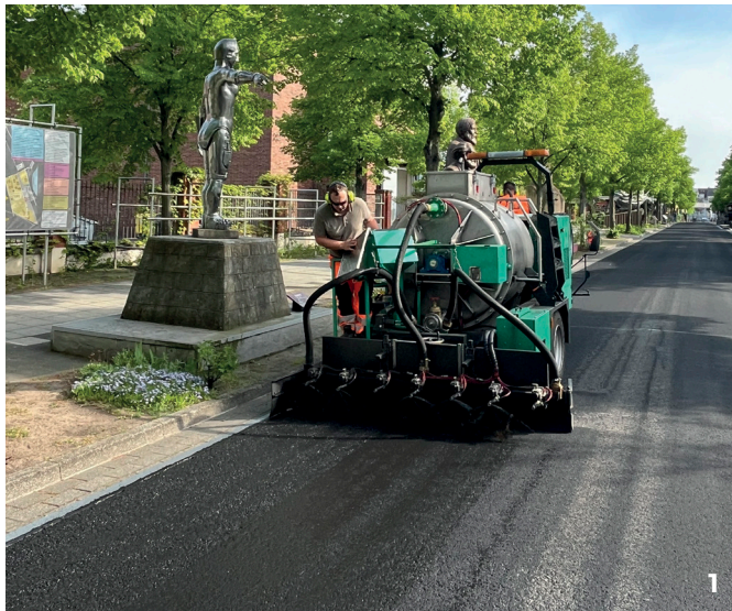
1 Onyx application | 2 finished surface | 3 Nozzle spraying device
